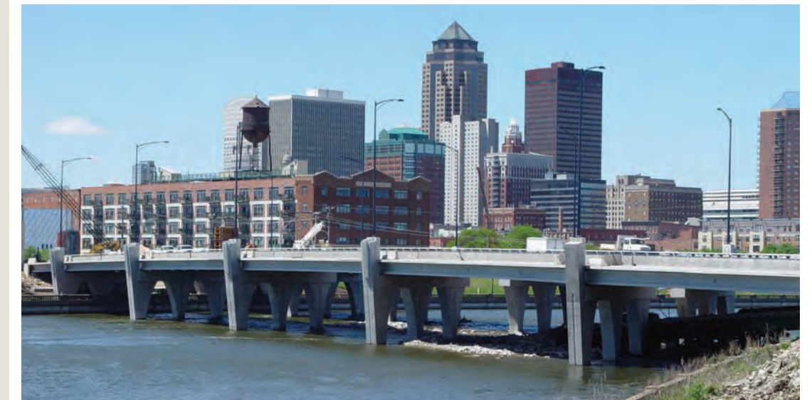
Construction of SE Connector Bridges Nearing Completion
