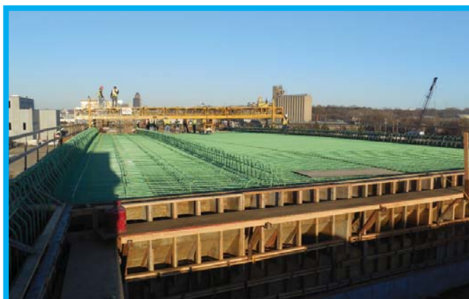
Bridge over UPRR
