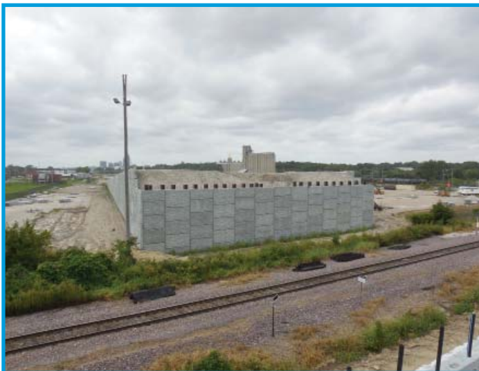
Mechanically Stabilized Earth (MSE) Walls at Union Pacific Railroad
