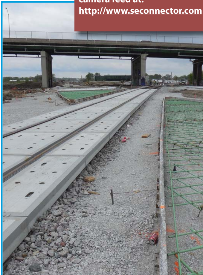
Railroad crossing beneath SE 14th Street
