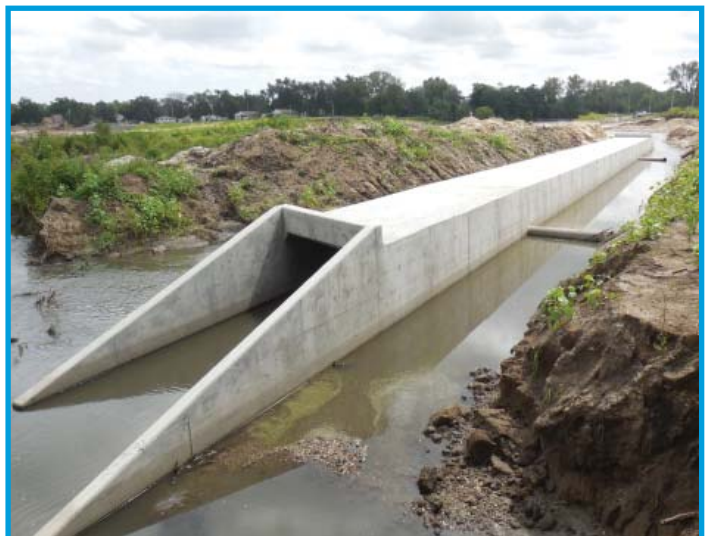
140-foot Reinforced Concrete Box Culvert (RCBC) in Dean's Lake
